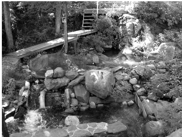
Fig. 2. Fish ladder and resting pools for alewives along the Damariscotta River (Maine). Photo by Barry Rodrigue, 2009
