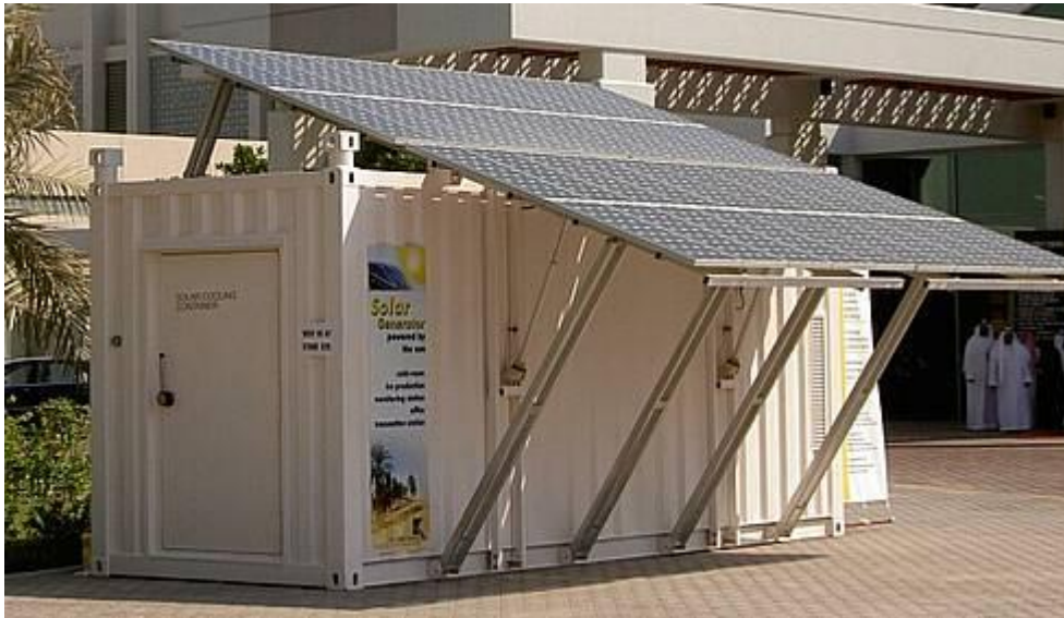
Figure 3 A solar-powered shipping container
